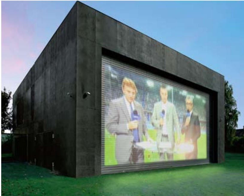
Closed mode: concrete panels and roller doors seal all the windows and entrances until the house looks like an impregnable concrete cube which does not disclose its identity.
