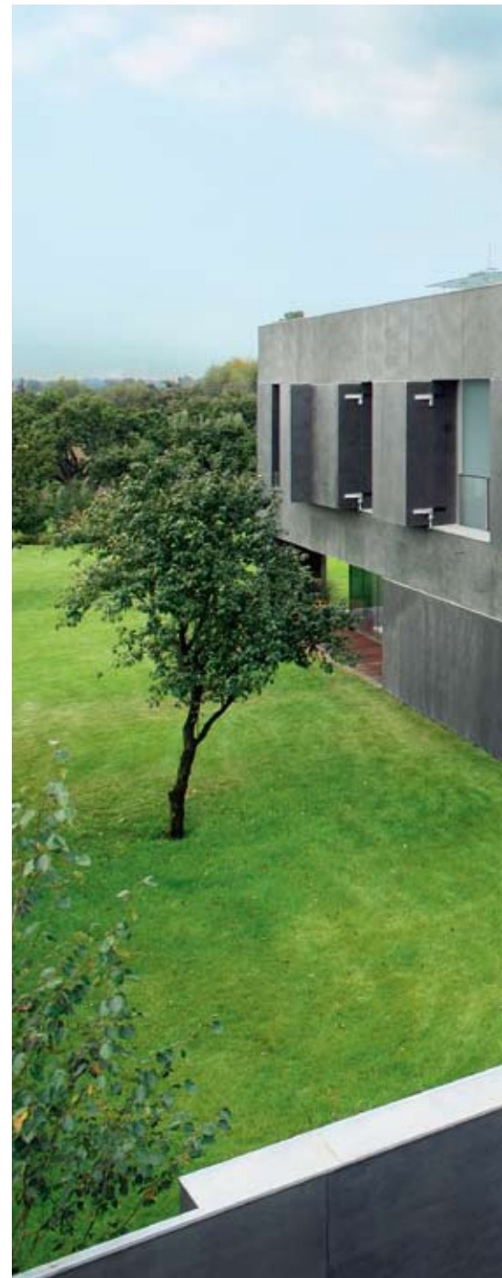
Closed mode: concrete panels and roller doors seal all the windows and entrances until the house looks like an impregnable concrete cube which does not disclose its identity.
